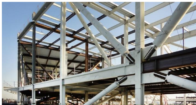
Fig. 14.4 Addition of Steel bracings
