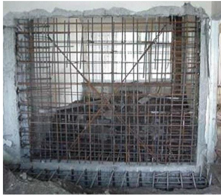
Fig. 14.3 Addition of shear Wall
