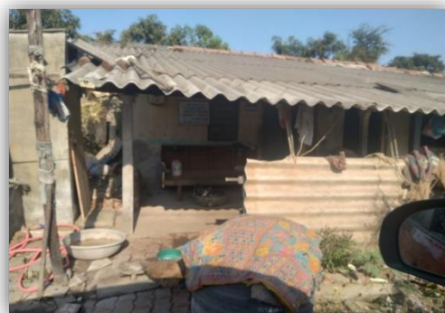
Fig. 4.8 House (Kewada Village)
