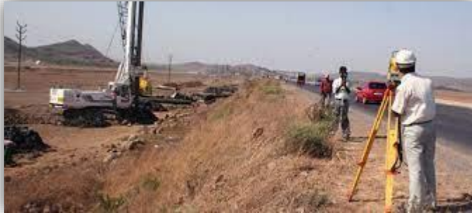
Fig. 5.3 Site investigation and surveying
