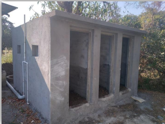
Fig. 4.6 Public toilet under construction (Kewada Village)
